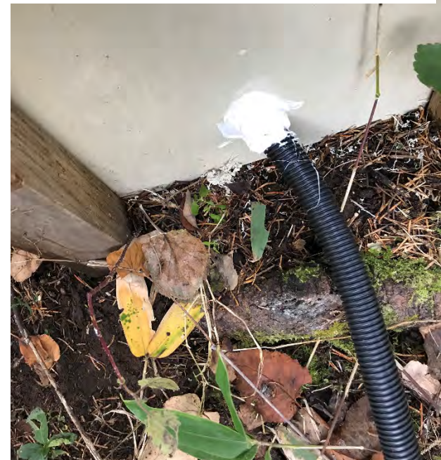
200mケーブルはパイプに入れてネズミを避ける The 200 cable was put into a plastic pipe to avoid animal bites
