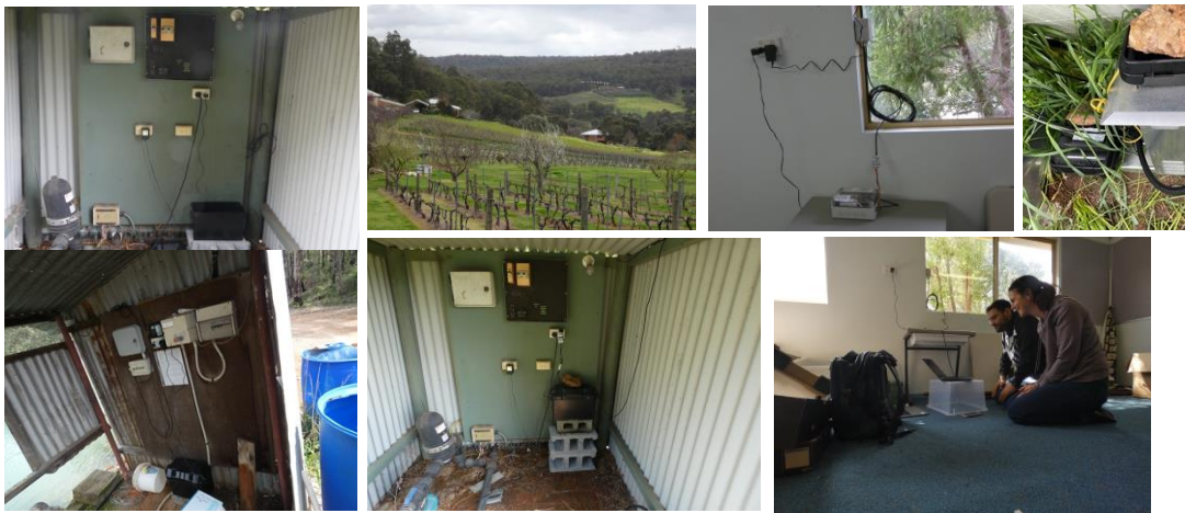
Fig. (2) Deploying the infrasound sensors in Perth array sites and Katanning site.
