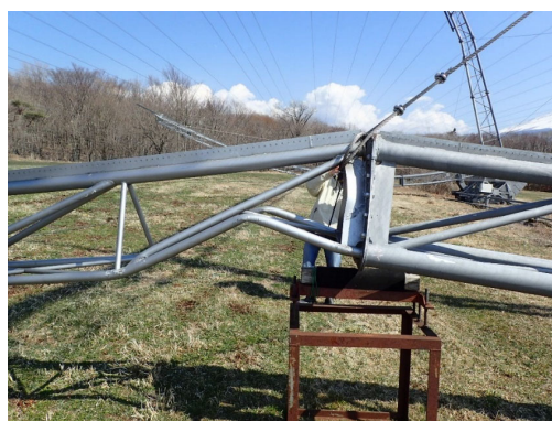
Broken Fuji antenna structure in March 2019.
