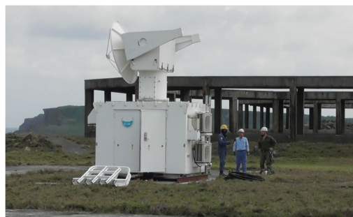
Ka-band radar installed on Yonagunijima.
