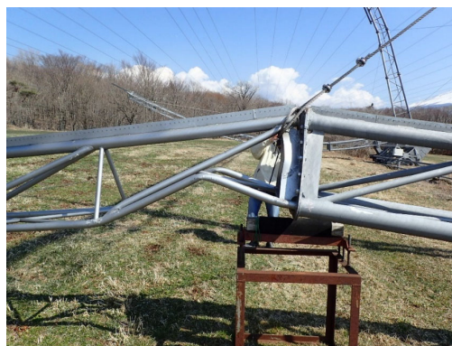
Broken Fuji antenna structure in March 2019.
