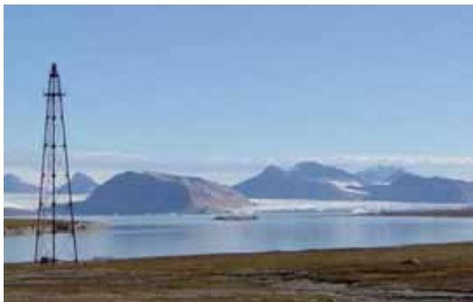
The airship mooring mast in Ny-Ålesund.
