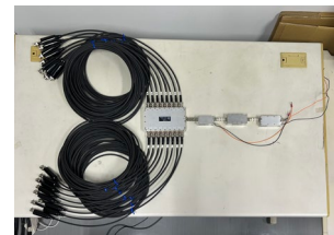
Configuration of the RX system, including a 16-port power combiner, two LNAs, and a BPF.
