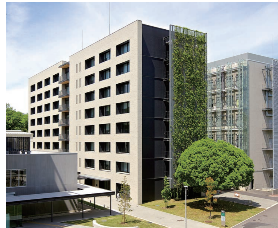
研究所共同館Ⅰ Research Institutes Building I
