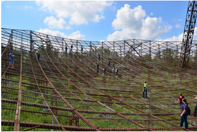
Figure 1. The main antenna of Kharkiv incoherent scatter radar (diameter 100 meters).
